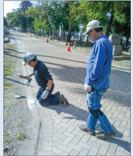
City workers installing the tiles at the Old City Cemetery.
