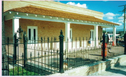
Heritage Museum after renovation
