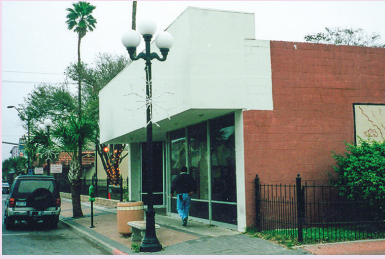
Facade of UETA building before renovation in 2002
